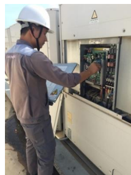
Air conditioning maintenance inspection
