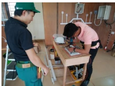
Power Distribution work
